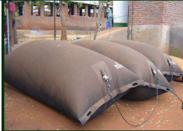
Biogas from the Flexigester® is stored in rubber gas bags for later use in the orphanage kitchen, providing a valuable alternative fuel source.
